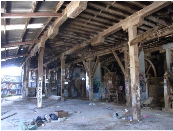
2011: Ground floor interior Building 5 showing massive timber structure and row of brick presses
