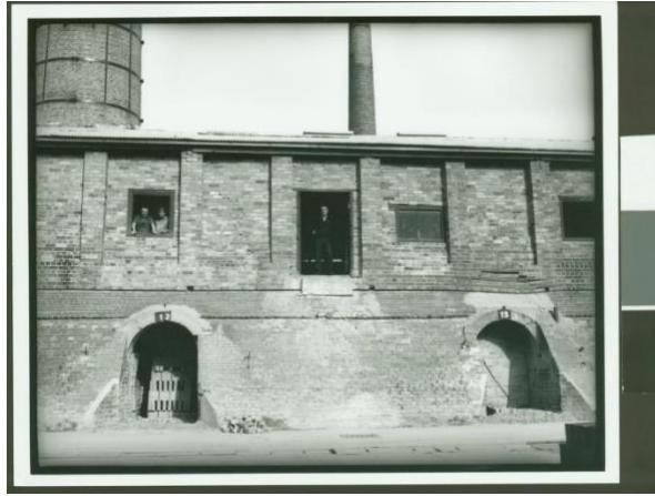
Prior to closure: Kiln showing workers on upper level and bricks stacked into the firing chamber (Source: Grant Hobson, SLV Collection)
