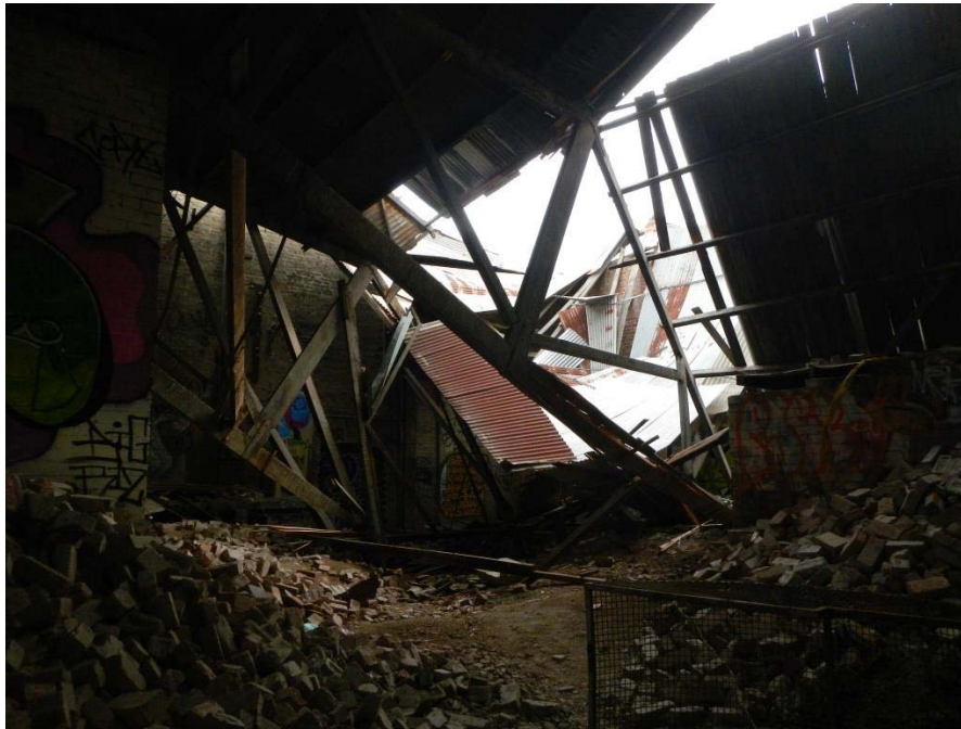
Figure 2 The former Engine House showing the damage caused by the collapse of the roof.
