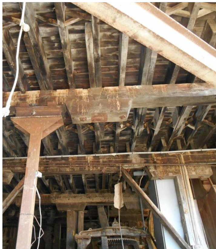
Figure A1-6 – Removal of timber post below remaining timber corbel. Spliced end of floor beams are no longer supported. Beyond, failure of timber corbel.
