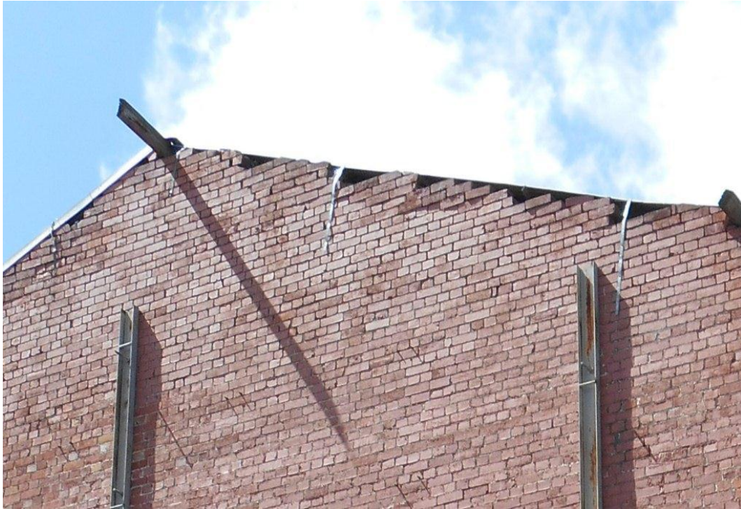
Figure A1-15 – Detail of damaged and unstable bricks along western wall.
