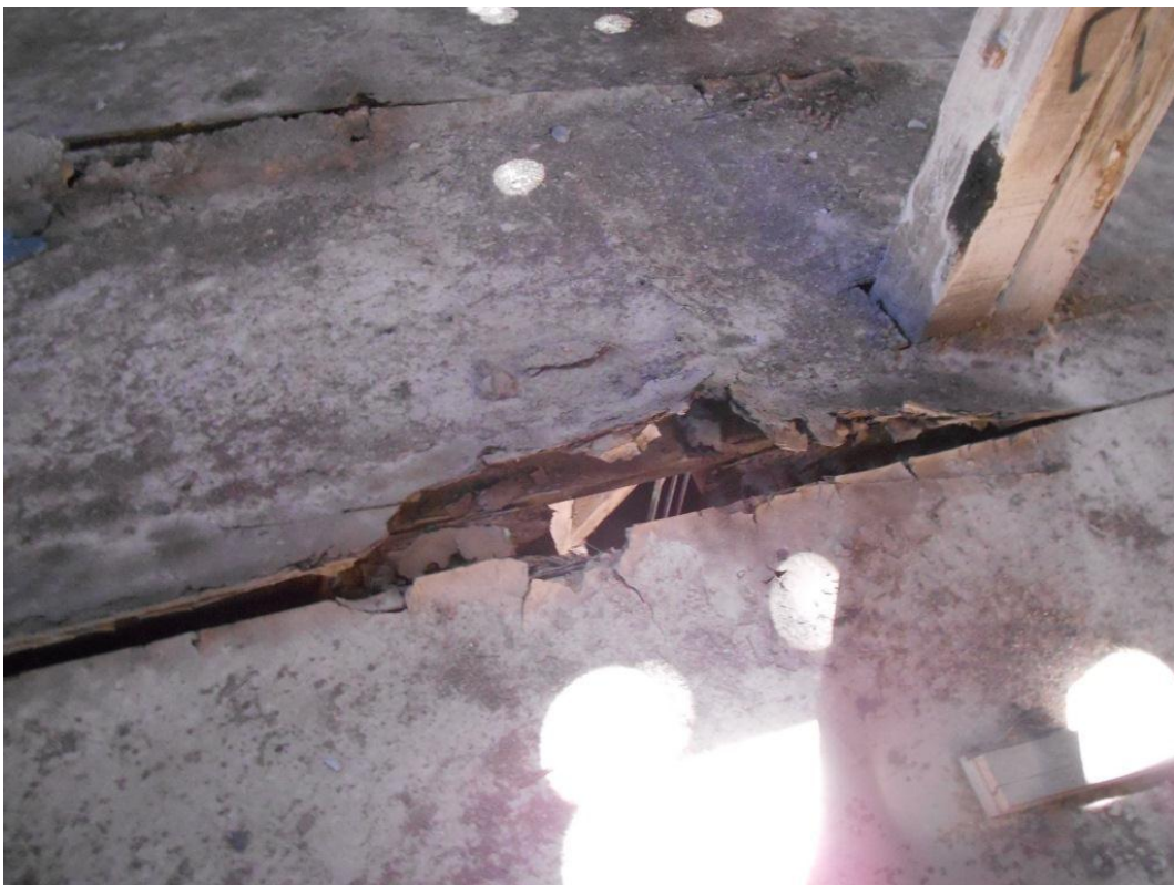
Figure A1-10 – Local collapse of timber flooring
