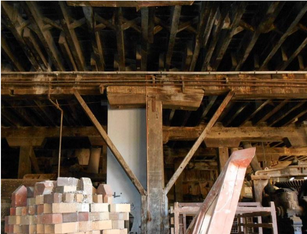
Figure A1-9 – Failure of column capital
