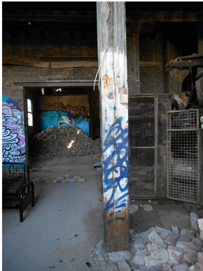
Figure A1-8 – Vertical splitting of timber posts.
