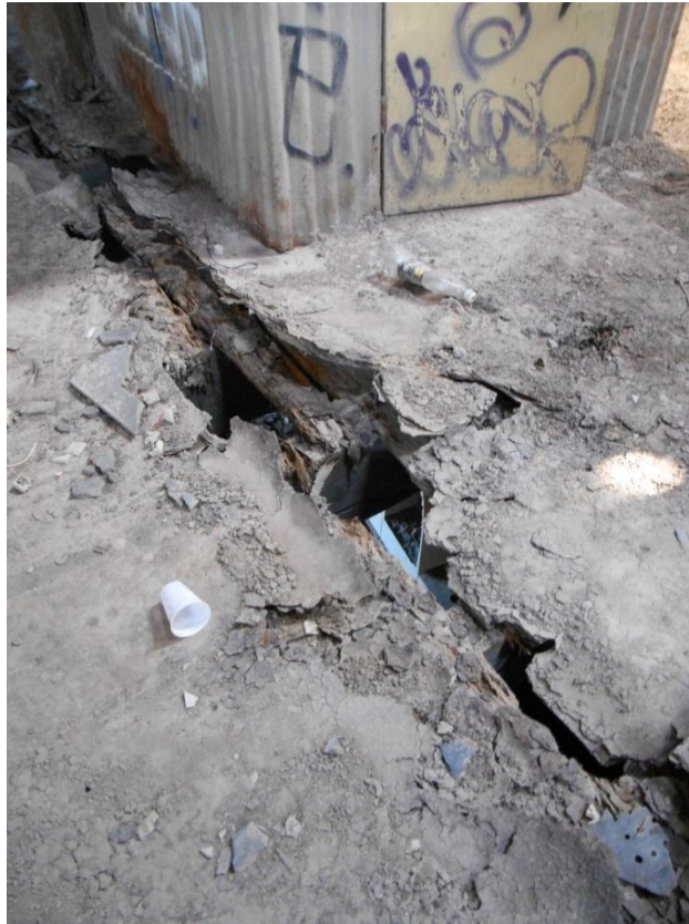
Figure A1-11 – Decay and collapse of timber floor and lining.
