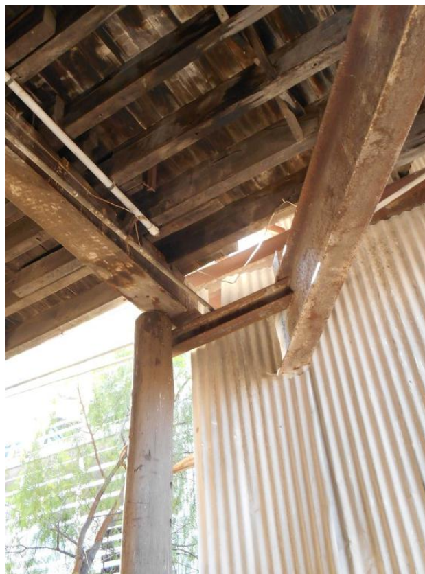
Figure A1-4 – Displaced supplementary timber post beneath timber floor beam
