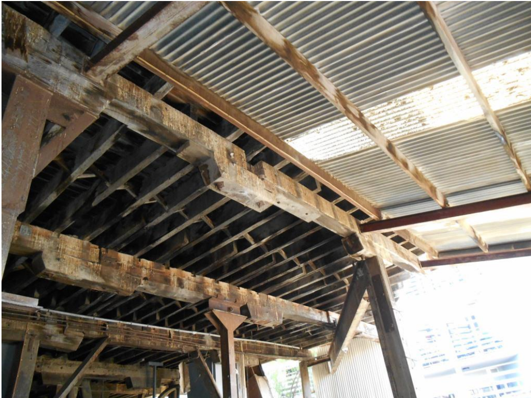
Figure A1-7 – Horizontal splitting of inadequately supported timber floor beams.
