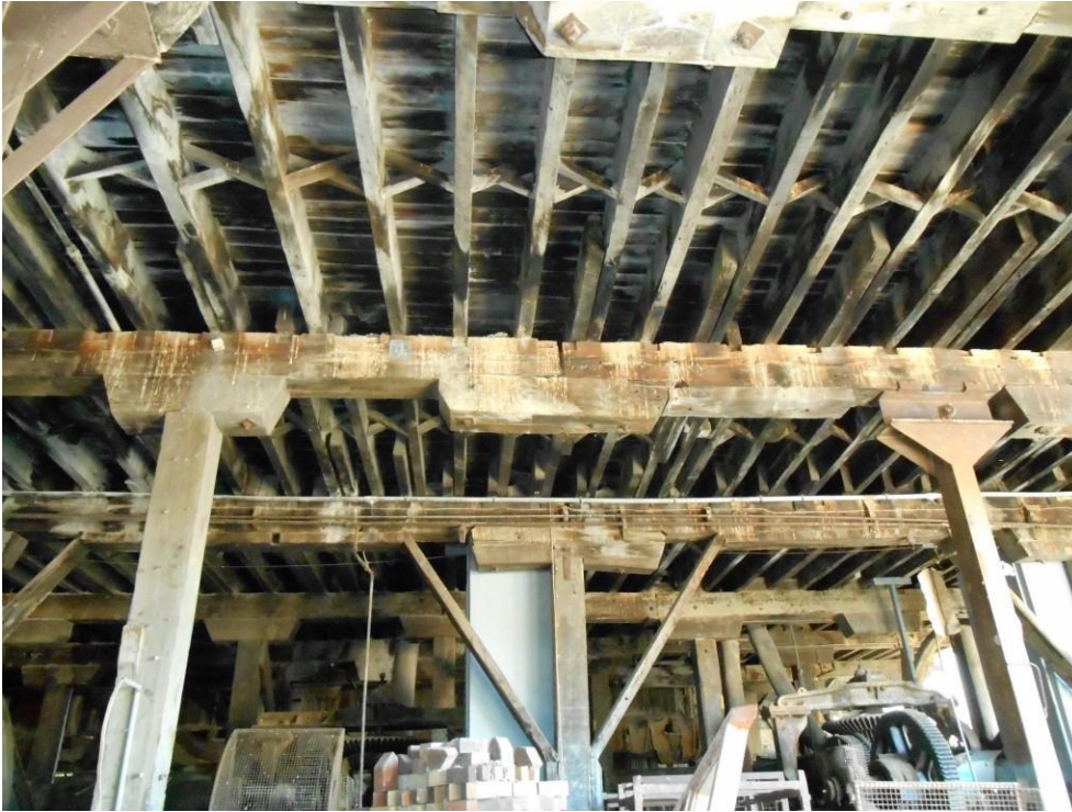
Figure A1-5 – Removal of timber post below remaining timber corbel. Free end of floor beams are no longer supported. Beyond, failure of timber corbel.
