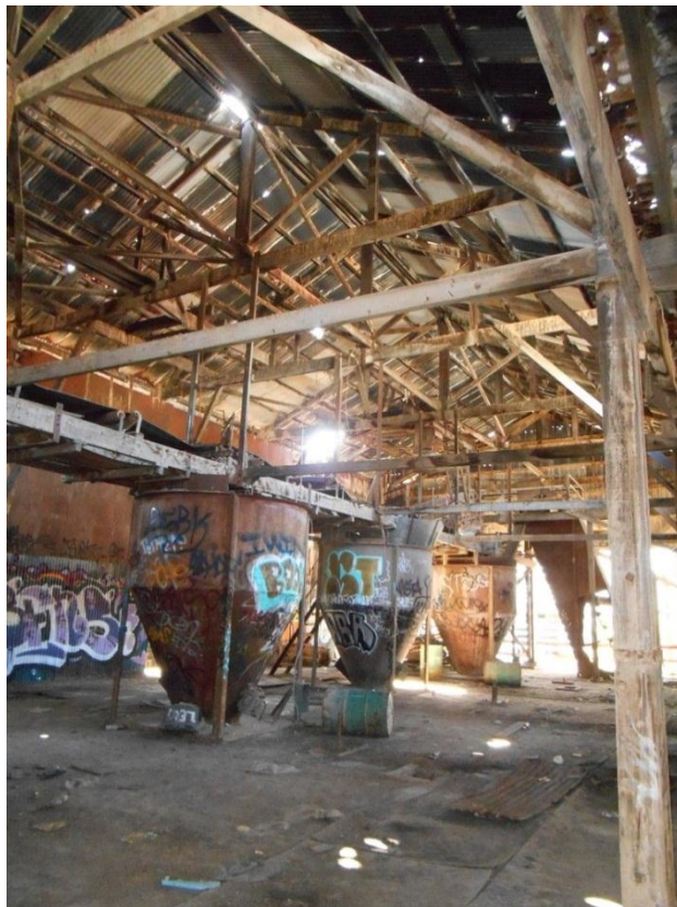
Figure A1-12 – Timber trusses and framing at roof level.
