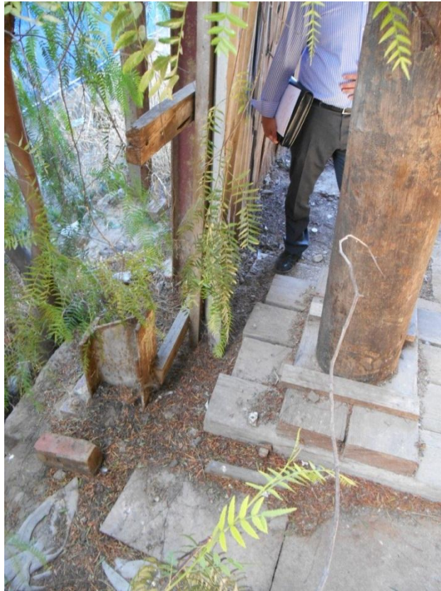
Figure A1-3 – Remnant section of steel post and timber sleeper support of supplementary post
