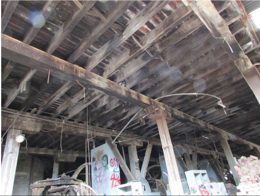
Building 5 First floor framing. Discoloration of timber from prolonged exposure to ingress of water. Top edge of timber rotted to a depth of 25-30 mm in the places available to be inspected . Ad-hoc structural repairs.
