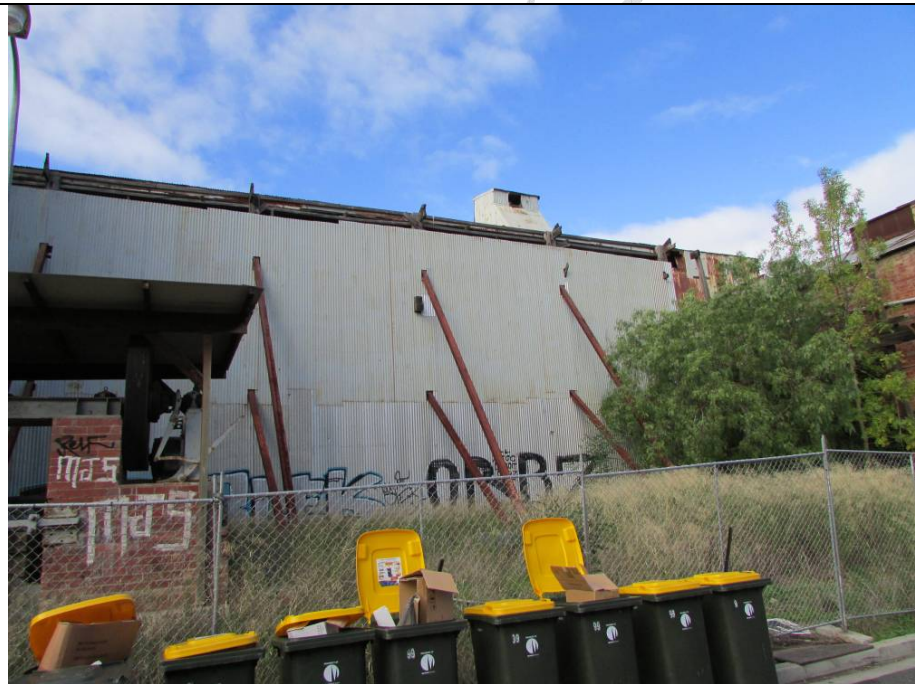
Building 5 – Western Annex external steel bracing frames View from Brickworks Drive
