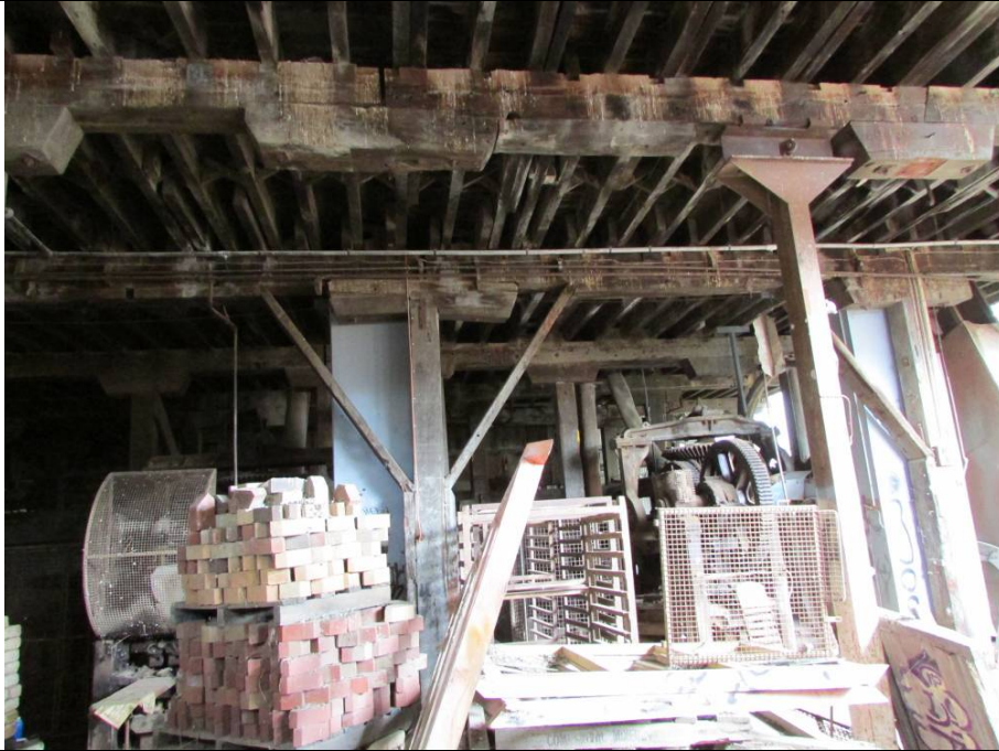
Building 5 – First Floor framing. Past practices associated with altering framing to accommodate the industrial function of the building. The majority of these construction practices, with rudimentary and agricultural are structurally sound
