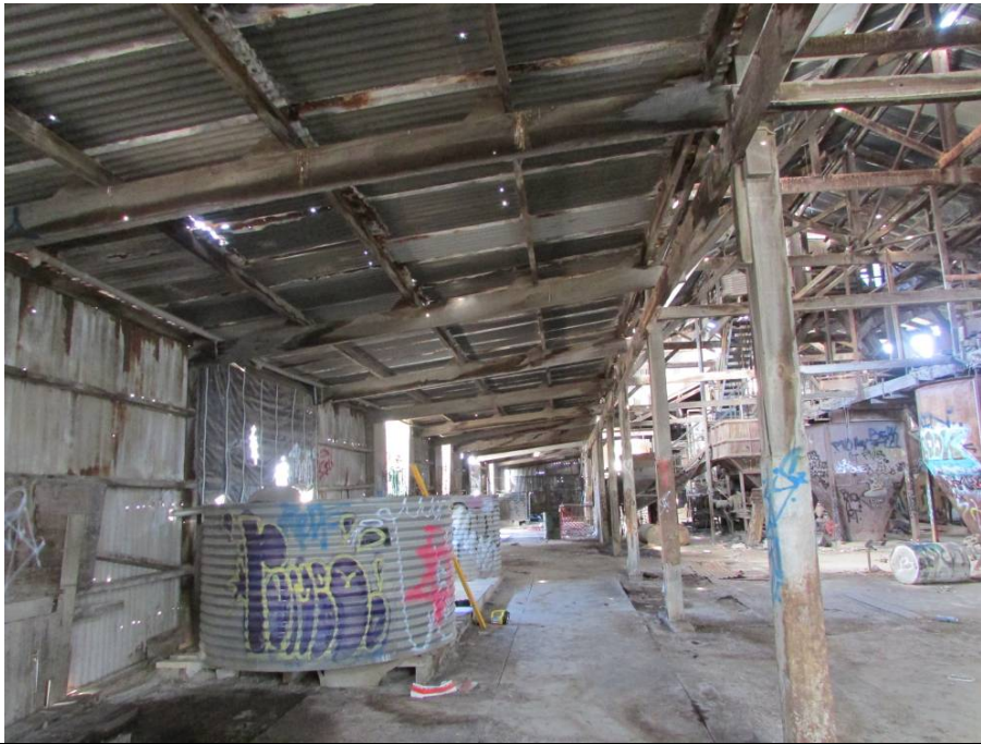
Building 5 – Lower Roof – East Wall Looking South Note the water tanks , approximately 1.2m deep. Representing a potential load on the floor of 12 kPa. This may explain the crushed timber capitals under . Residential floor loads are 1.5 Kpa, Office floor loads are 3.0Kpa
