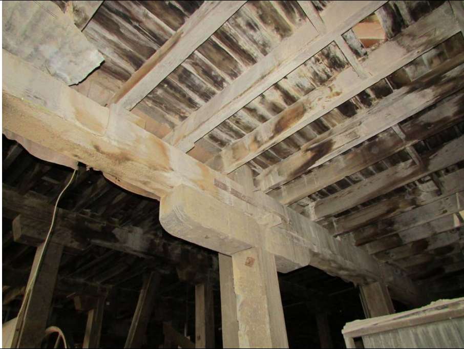
Building 5 – Western Annex. Eastern Edge . Floor joist and other timber properties seem to be sound
