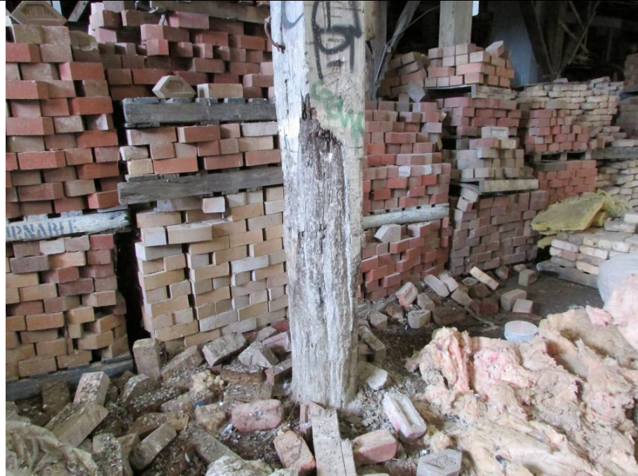
Building 5 First floor framing – Post base. I suspect that this damage is mechanical associated with the movement of materials in the industrial processes of the buildings historical context . Exposed timber is sound and in good conditions
