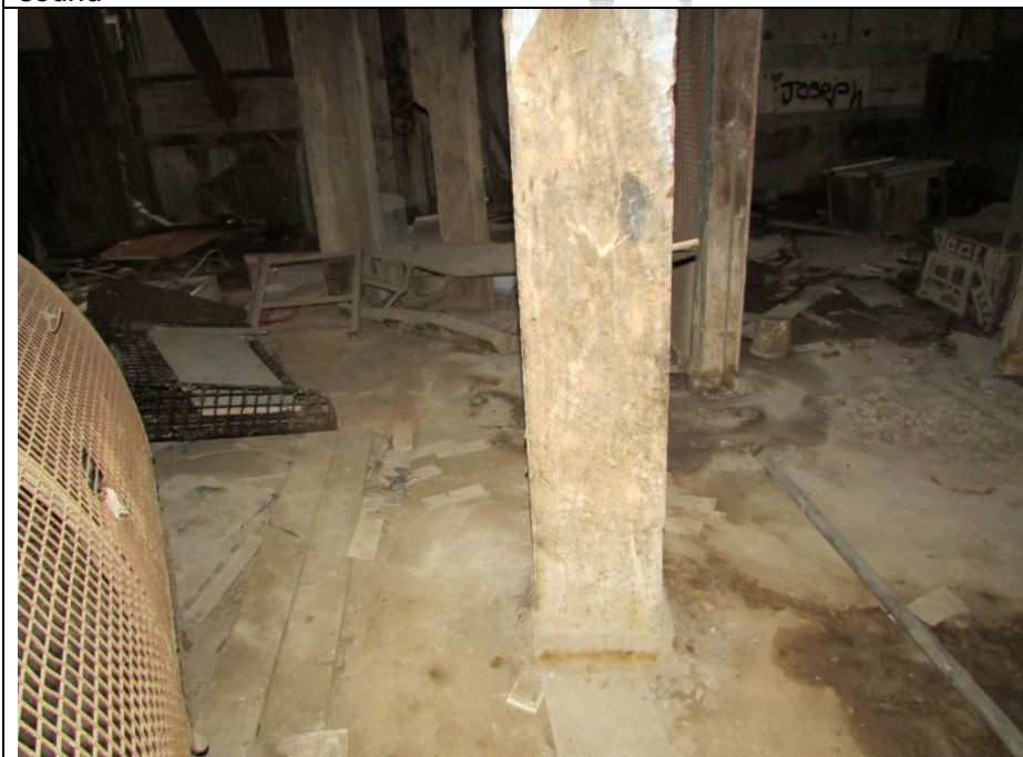
Building 5 First floor framing posts in the western portion of the building near the pressing machinery. This type of construction is consistent with the posts cantilevering to provide structural lateral stability for the building. Post base is sound and in good condition
