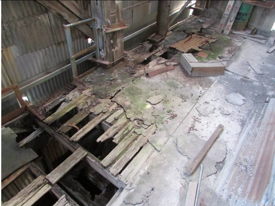
Building 5 Western Annex- Flooring badly affected by ingress of water and adverse affects of water over a prolonged period of time and is condemned as structurally unsound
