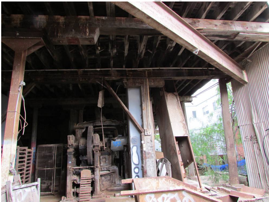
Building 5 First floor framing ad-hoc construction practices. The steel beam is supported by a steel column behind the CI sheeting. The circular post is poor construction practice. This type of poor construction practices affects no more than 10 % of the first floor area.
