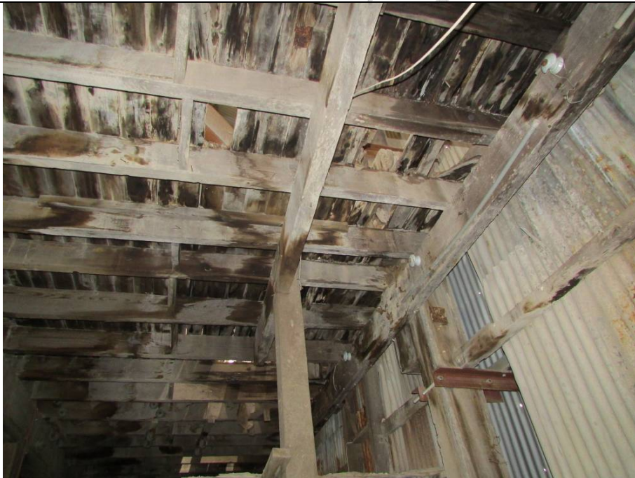
Building 5 – Western Annex – Western Edge . The majority of the section still appears to be sound. This framing is not condemned until additional investigation is undertaken to determine the depths of the top edge surface rot.
