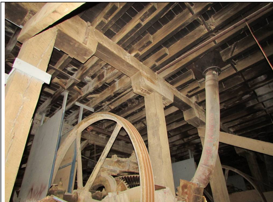
Building 5 – First floor framing over the pressing machinery in the Western portion of the Bld 5. Columns, capitals, beams and floor joist are all in good condition. I suspect also that the flooring is in reasonable condition given the environment that is subject to. Fundamentally the 'structure' is sound
