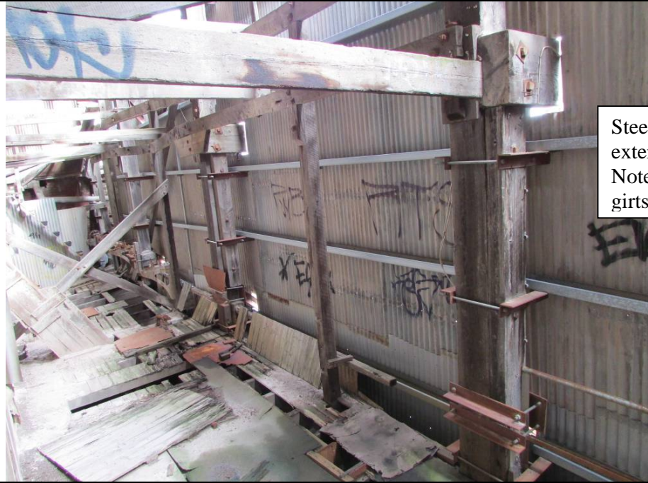
Building 5 – Western Annex- Internal – Note bracing connections. The floor of the western annex is lower than Building 5 by approximately 1500mm
