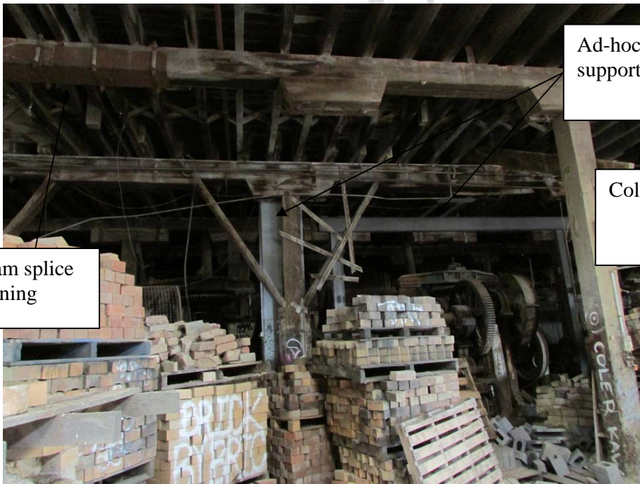
Building 5 First Floor framing. – Typical examples of poor building and construction practices within the building. These types of practises affect approximately 10 – 15 % of the first floor framing . But it also demonstrates that past practices have intended not to overload the existing/original timber framing
