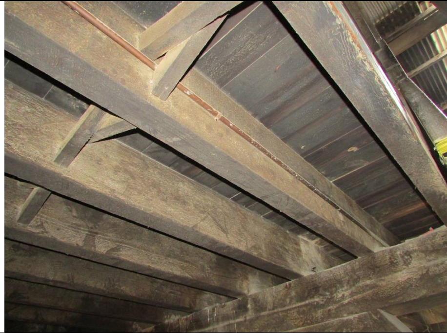
Building 5 – Typical first floor framing condition for majority of the floor. Water ingress has in areas had a detrimental affect on the floor joists
