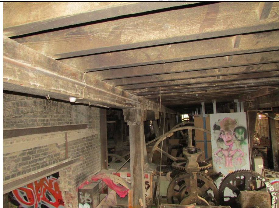
Building 5 – First floor framing looking North. 75- 85 % of the floor framing is in this conditions
