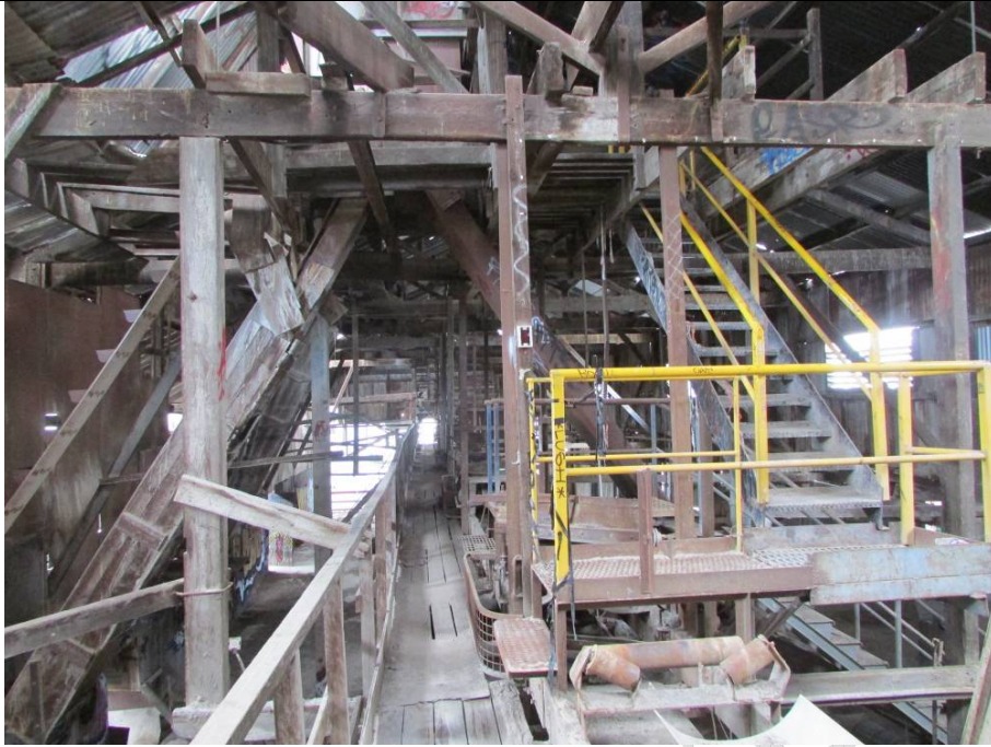
Roof Building 5 – Typical ad-hoc retrofitted mezzanine type industrial access framing, walkways and machinery supports
