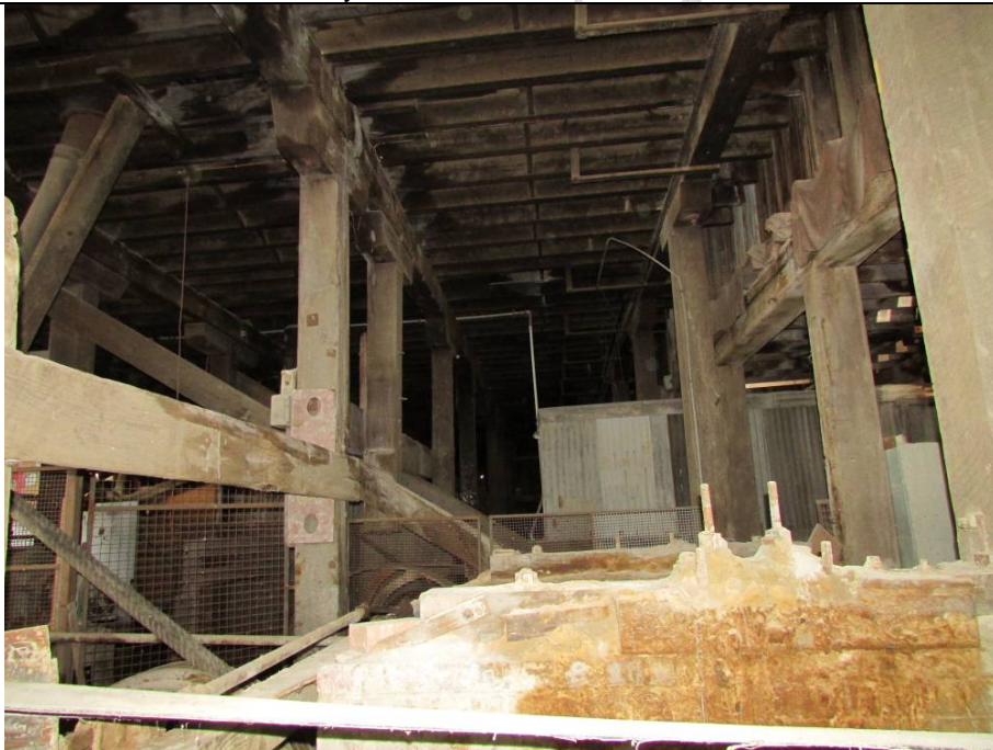
Building 5 – Western Annex- Note construction of step between the floor of Building 5 and the lower floor of the western annex
