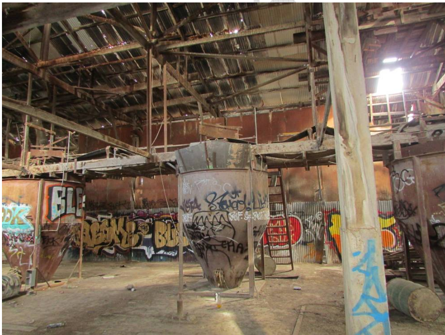
Floor Building 5 – Typical ad-hoc retrofitted mezzanine type industrial process access framing and hopper supports
